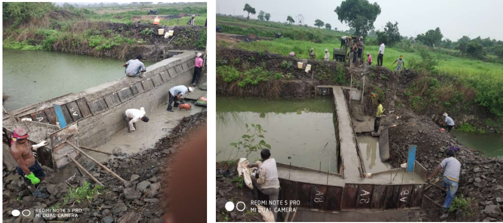
Construction of a Cement Nala Bandh as part of MRG Consultant's CSR initiatives.
